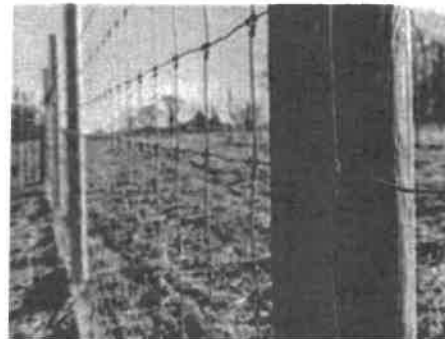
Wildlife-friendly barb/smooth wire fence. This is Wildlife-friendly wire woven fence a permeable fence.
